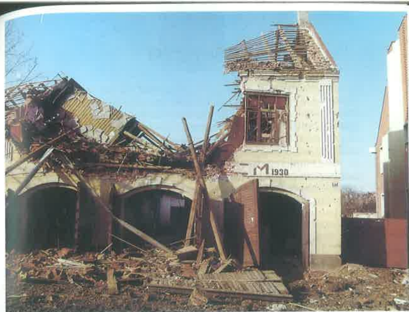
Vinkovci, Nuštar, fire station, after destruction photo - personal property
