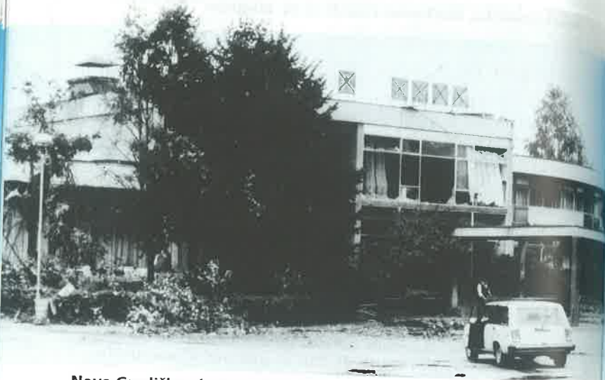
Nova Gradiška, destroyed motel next to the highway Zagreb - Belgrade
