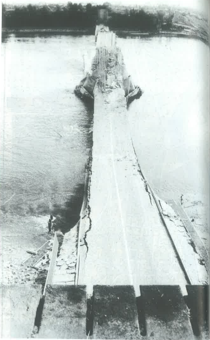
Županja, collapsed bridge Županja - Orašje, photo Nikolić
