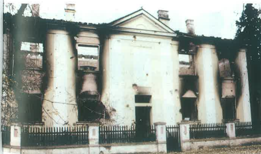
Osijek, apartment building, Car Hadrijan Street, photo Gregić
