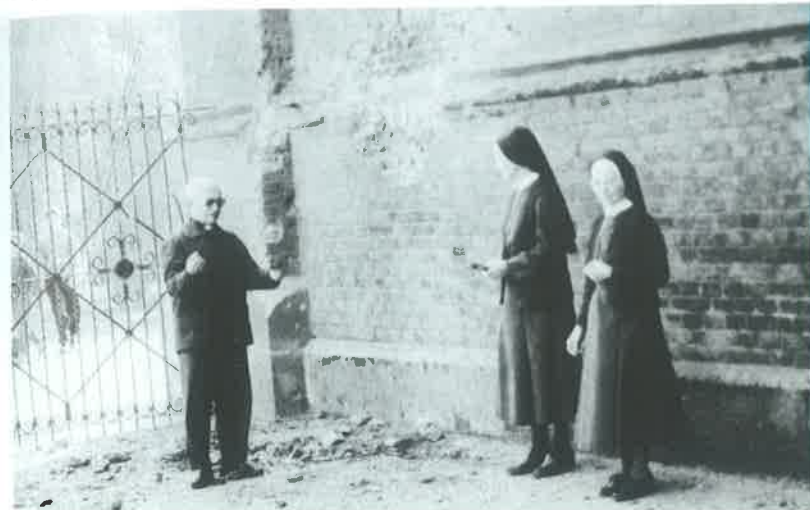
Đakovo, Cathedral, after damage, photo - personal property
