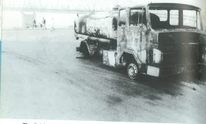
The Bridge between Slavonki and Bosanski Brod,
