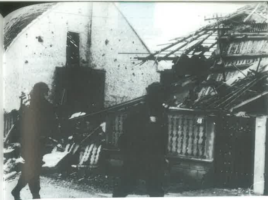
Vinkovci, Mala Bosna (housing project)
