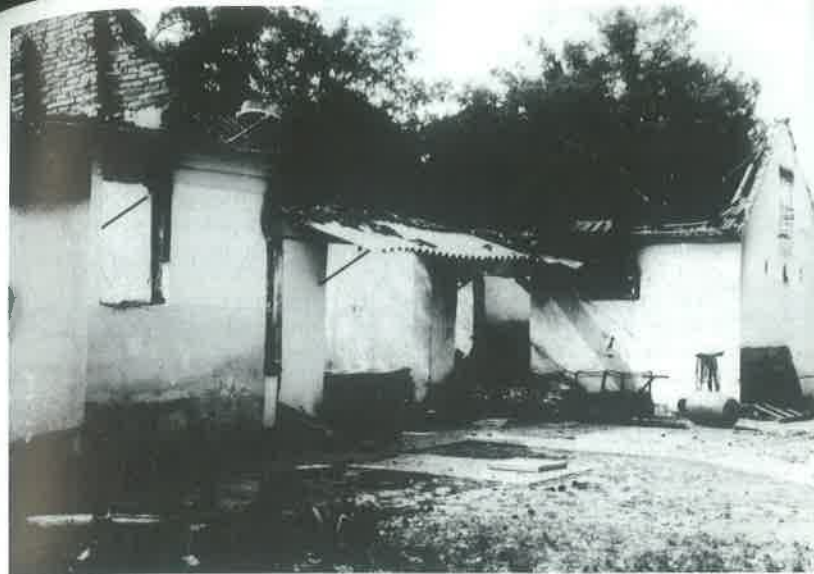
Vukovar, Čelije, 7-10 May 1991, completely destroyed and burnt village
