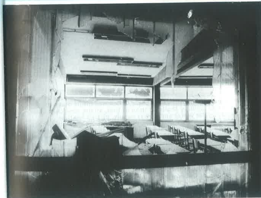
University of Osijek, Faculty of Civil Engineering
