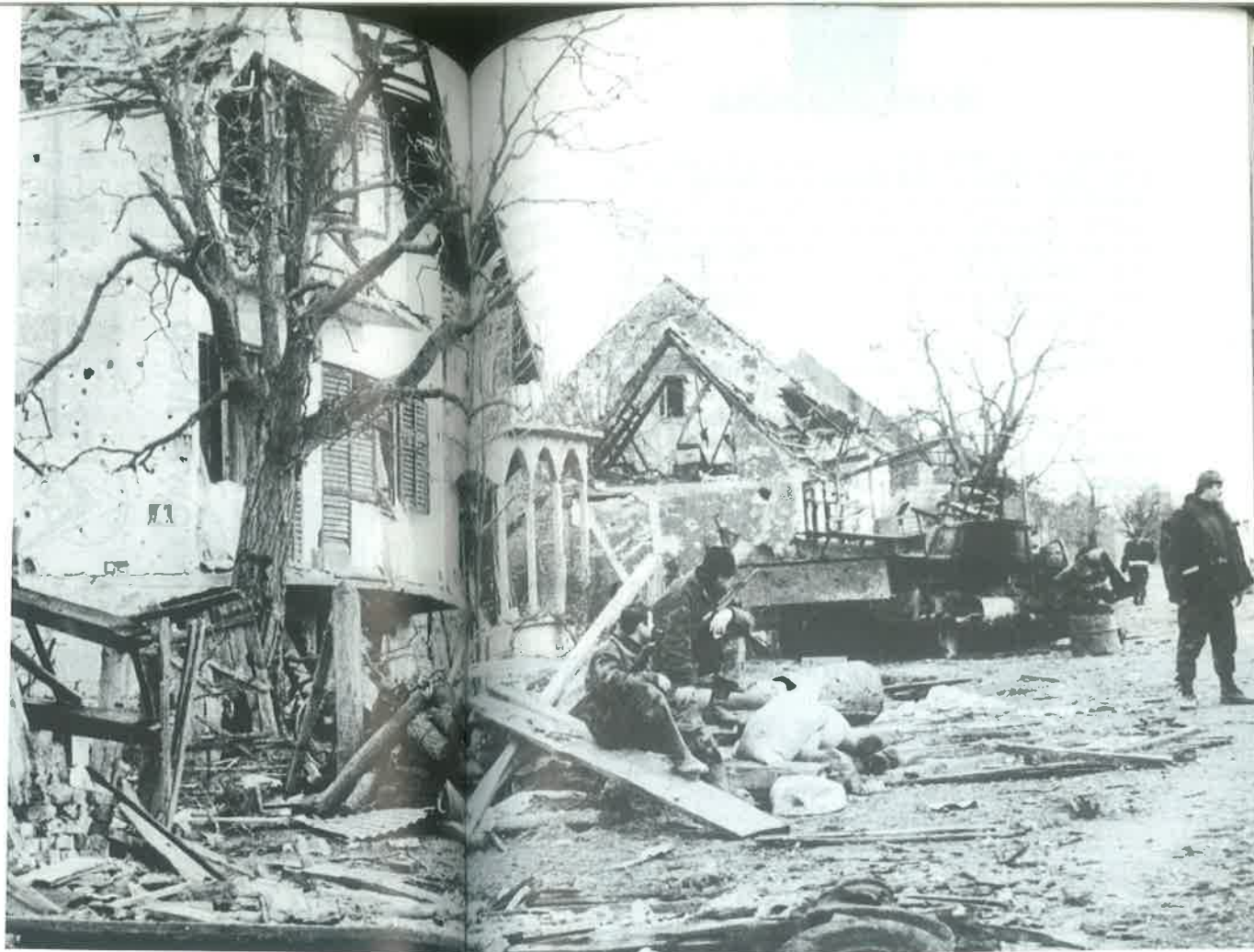
Nova Gradiška, scenes of destructions in commune Nova Gradiška
