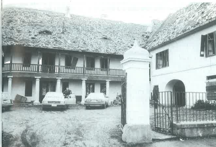
Vinkovci, Nuštar, Baroque castle Khuen - Belassi, after destruction, photo Smajić
