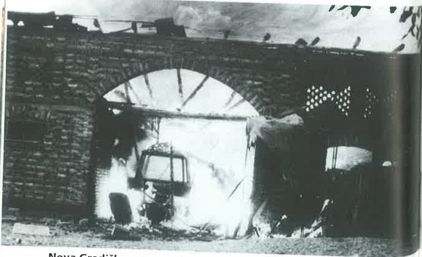
Nova Gradiška, scenes of destructions in commune Nova Gradiška 3
