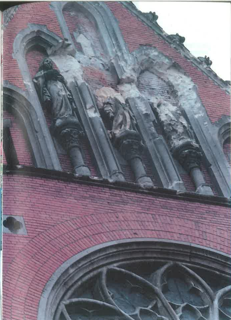
Osijek, parish church od St. Peter and Paul, photo Šimić
