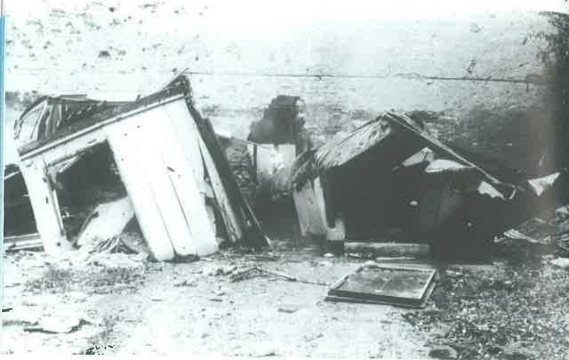
Nova Gradiška, scenes of destructions in commune Nova Gradiška 1
