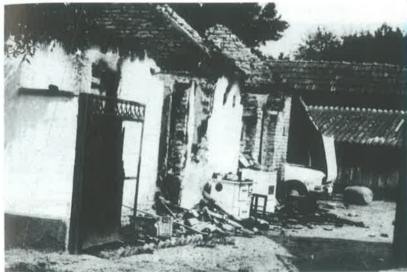
Vukovar, Čelije, 7-10 May 1991, completely destroyed and burnt village
