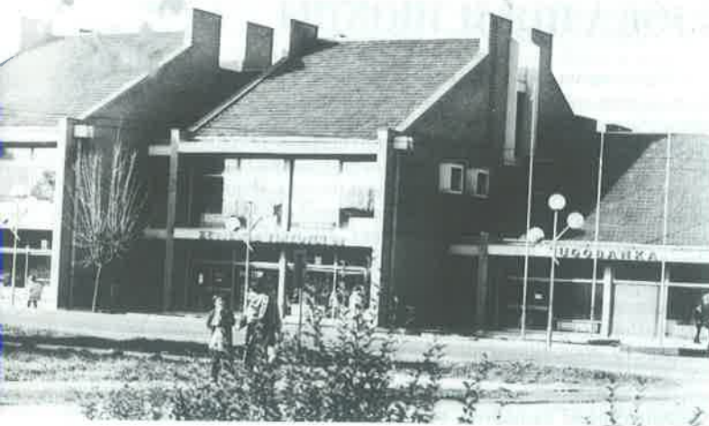
Vinkovci, Nuštar, shop "Zvijezda" Vinkovci, before destruction, photo Rubić
