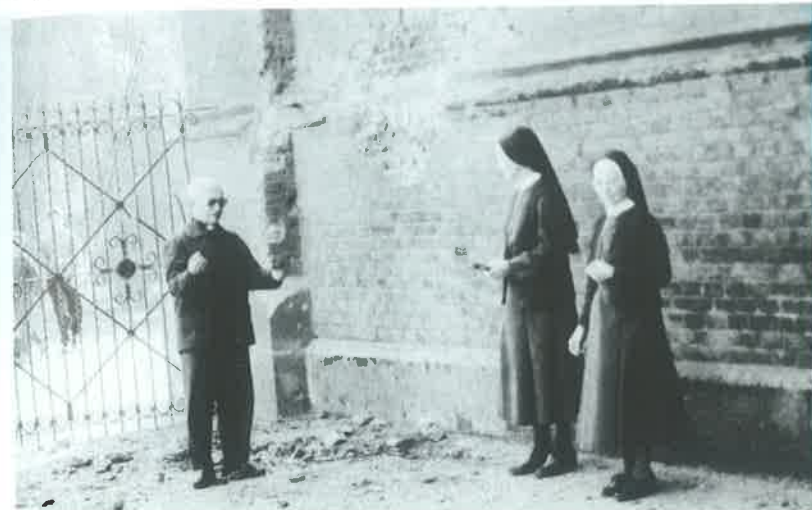
Đakovo, Cathedral, after damage, photo - personal property
